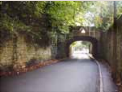
Walls & 1768 Bridge, Gledhow Lane
