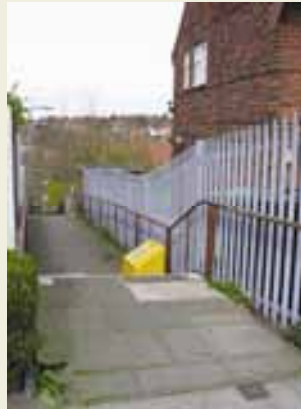
Galvanised steel industrial fencing along a path by houses detracts from the character of the area
