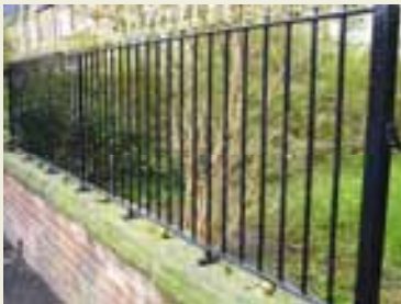
Good example of modern railings on an old wall
