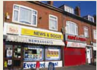
Clashing signs have a detrimental effect on the character of this parade
