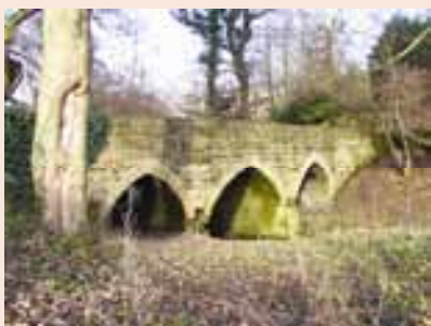
Bridge over Wyke Beck
