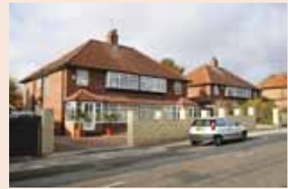
Wall-to-wall paving and unsympathetic boundary treatment
