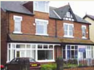
Replacement windows and new dormers should respect original design especially in semi-detached pairs and terraces
