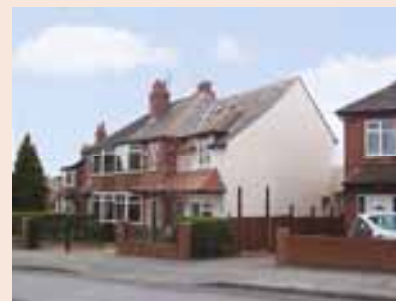
Western area - extending houses
