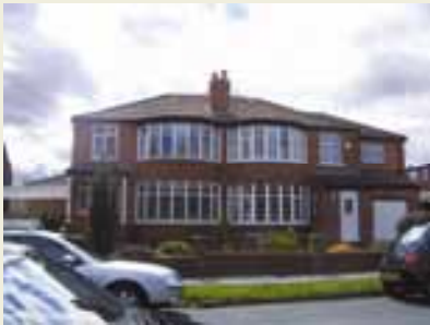
Good example of an extension which is in keeping with original semi-detached house on the left
