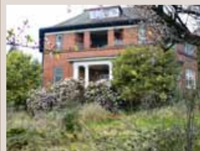
Theme 2: Neglected building on Oakwell Mount
