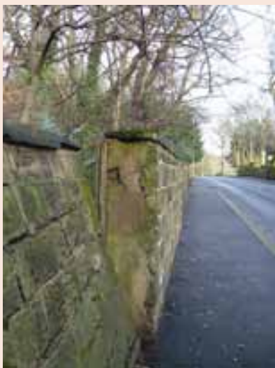
Wetherby Road stone wall in Conservation Area but in disrepair
