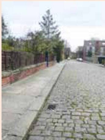
Yorkshire flags, stone setts and kerb, cast iron gully cover and original stone-capped boundary wall add character to street scene
