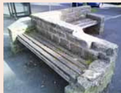
Seat in poor repair
