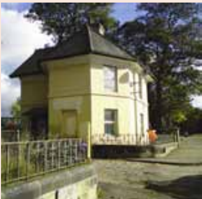
Moor Allerton Hall Lodge - a notable building and associated structures in disrepair
