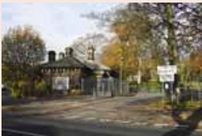
Lobb Cottage - derelict with incongruous fencing in Conservation Area
