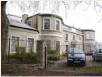
Moor Allerton Hall (Grade II listed)
