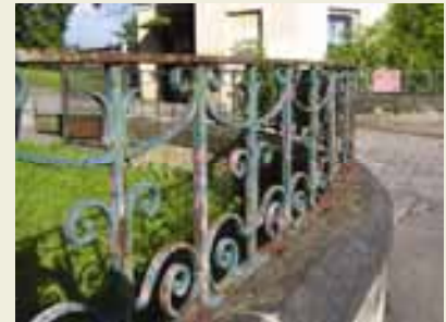
Historic iron railing in need of conservation
