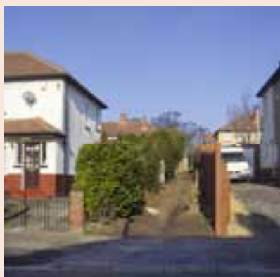
Ginnel in poor state of repair
