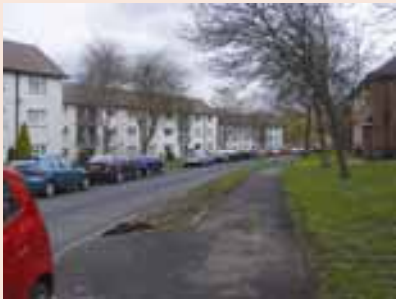
Grass verges eroded by parked vehicles
