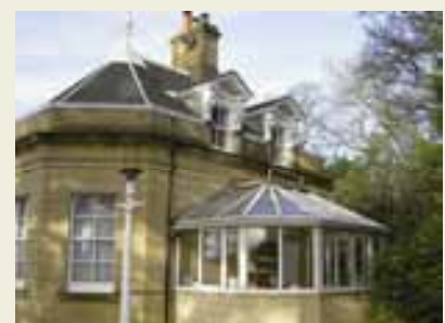
Attention to historic detail and care in the character of the addition
