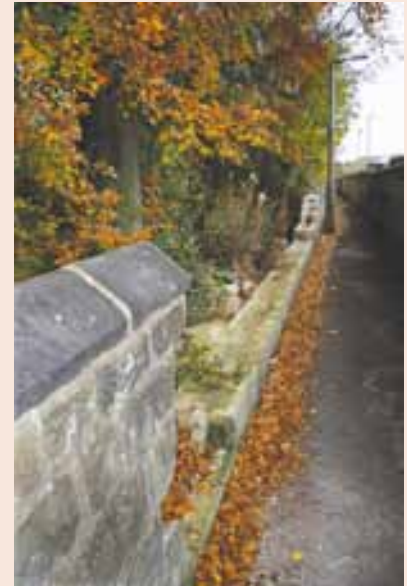
Historic ginnel wall being robbed of stone
